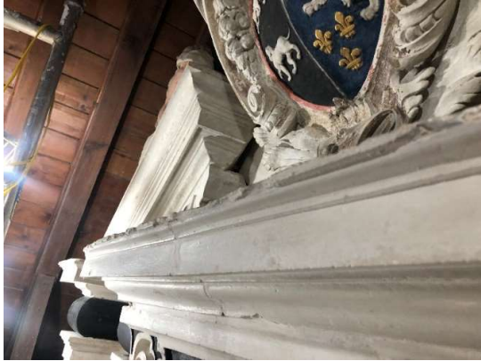
Figure 77 Central cornice (before repair)
