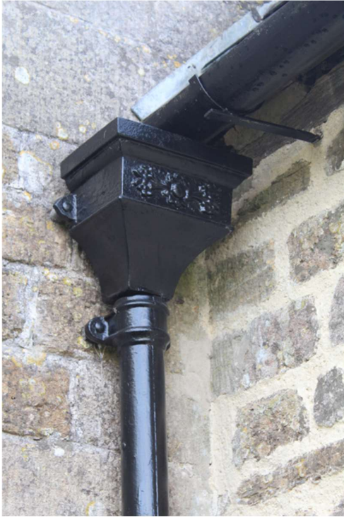
Figure 12 Painted rainwater goods
