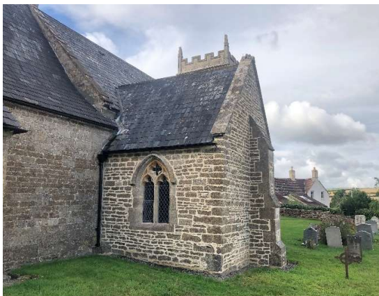
Figure 9 New pointing on the east wall
