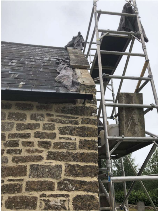
Figure 71 The east side copings being lifted
