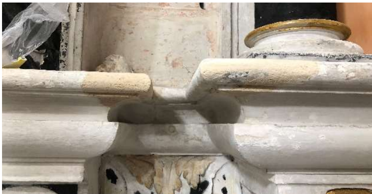
Figure 49 Completed repairs to the mantle
