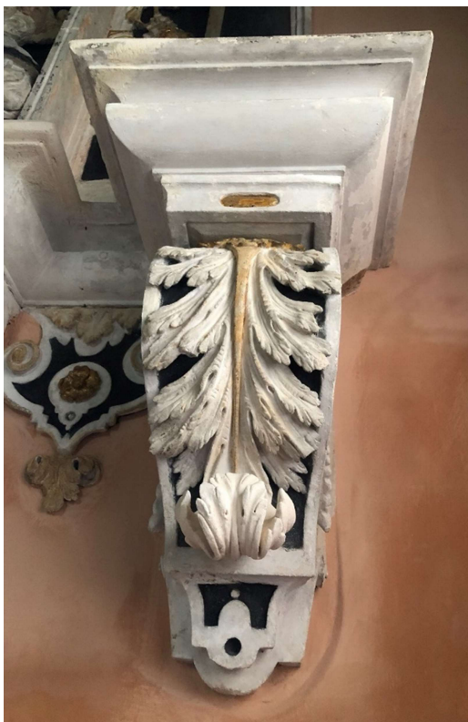
Figure 52 New carved leaf on the sinister corbel (face on)
