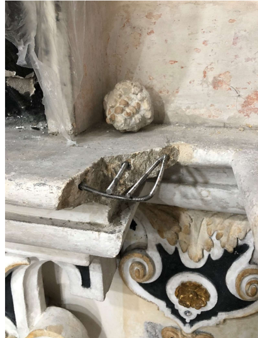
Figure 46 The stainless-steel armatures being installed to the sinister main mantle
