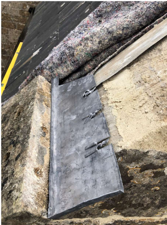
Figure 73 The lead tray before fitting
