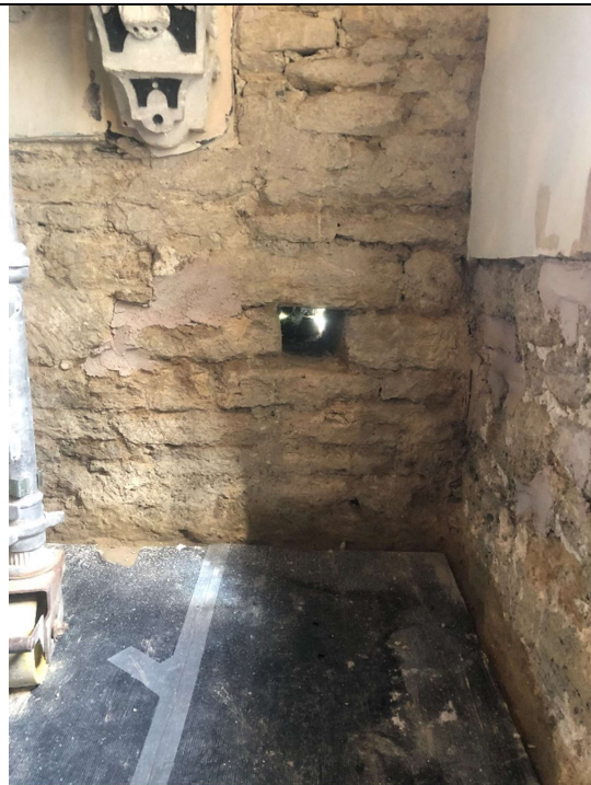
Figure 92 Interior north-east lower putlog hole
