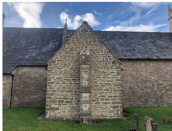
Figure 10 New pointing on the north wall
