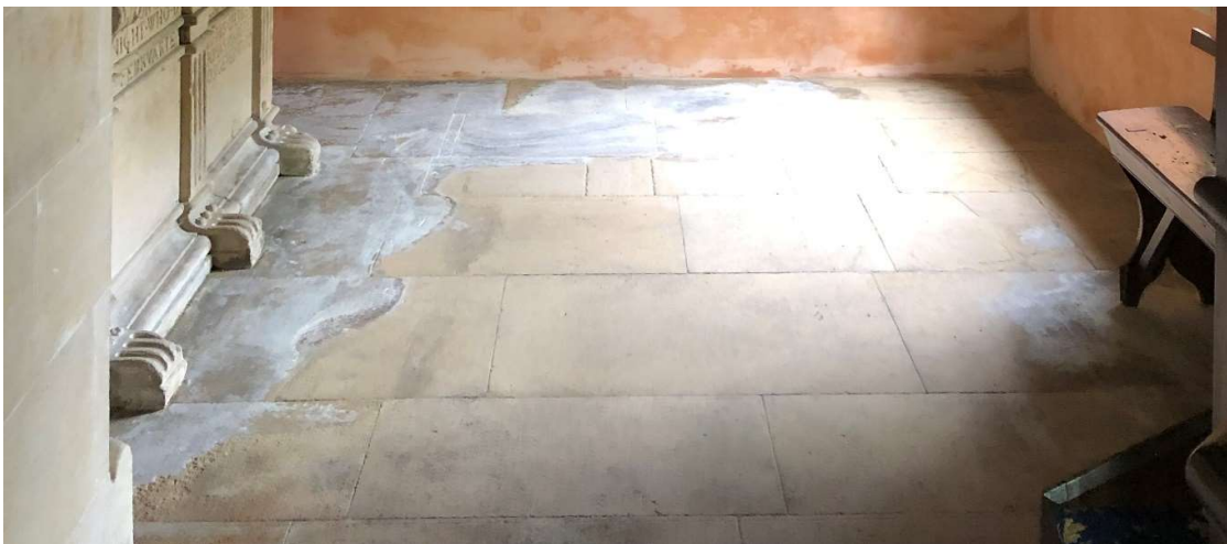
Figure 16 Horner Chapel floor after cleaning
