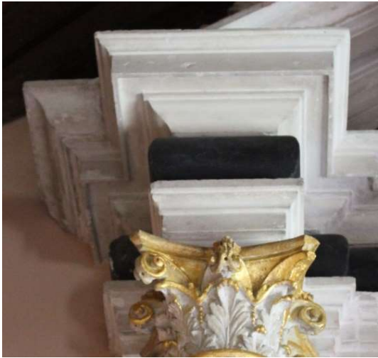
Figure 81 Dexter cornice (after repair)
