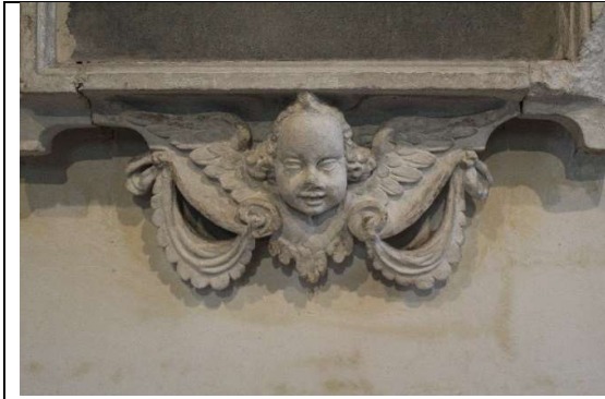
Figure 24 Before uplifting and limewashing the walls
