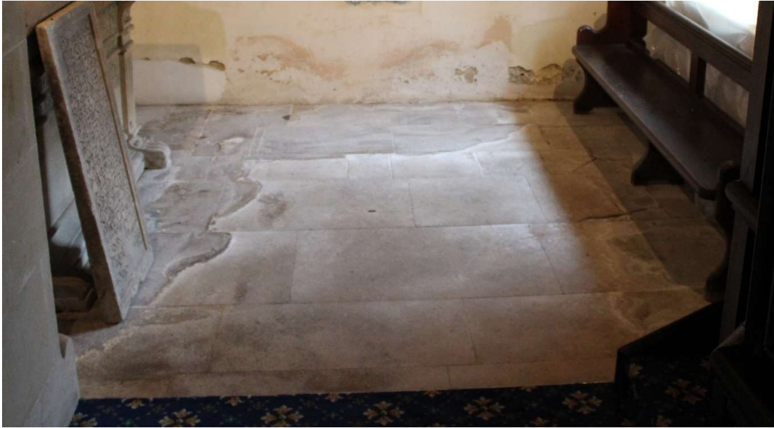
Figure 15 Horner Chapel floor before cleaning
