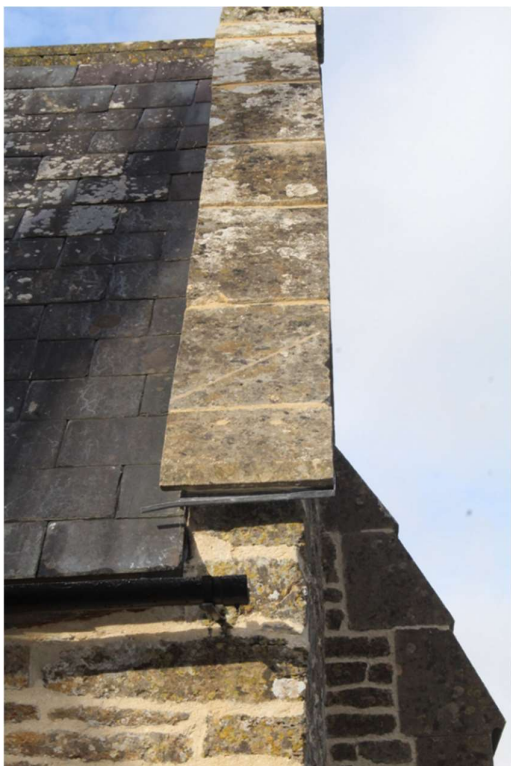
Figure 68 The east coping 45 degree cut in the dry
