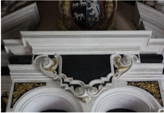
Figure 80 Central cornice (after repair)
