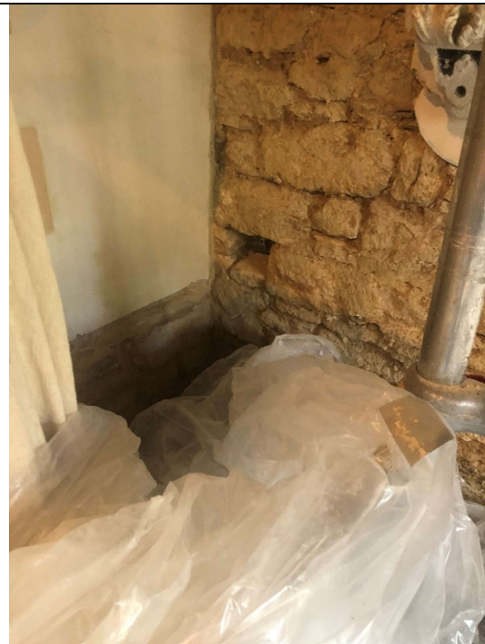
Figure 91 Interior north-west lower putlog hole
