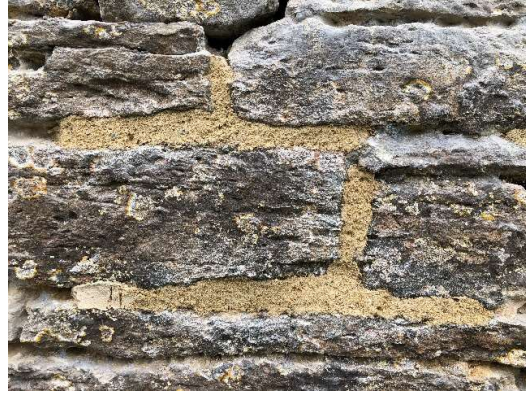
Figure 5 Mortar sample cool buff
