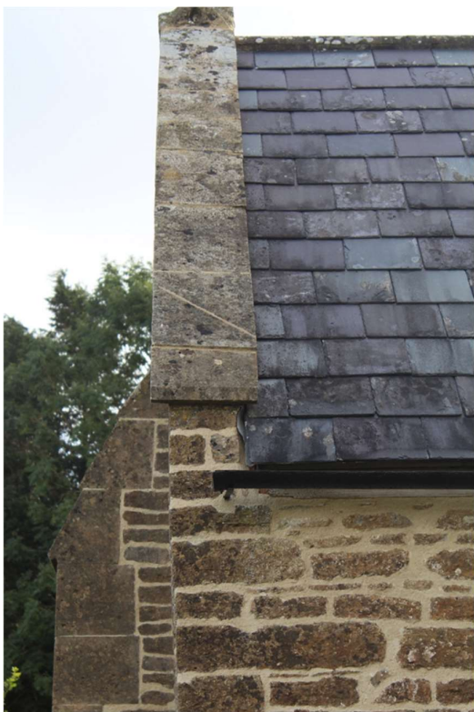
Figure 70 The east coping 45 degree cut
