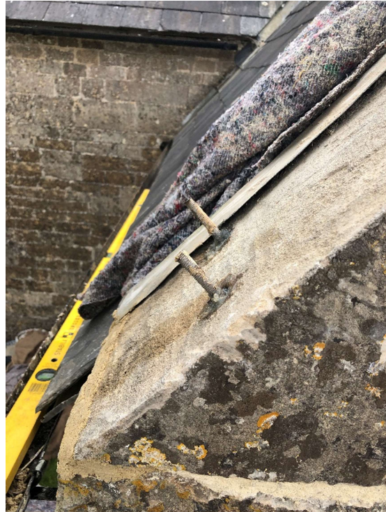
Figure 72 The new stainless-steel pins fitted
