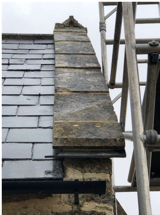
Figure 69 The east coping 45 degree cut in the wet; note how the coping is wetter above the cut.
