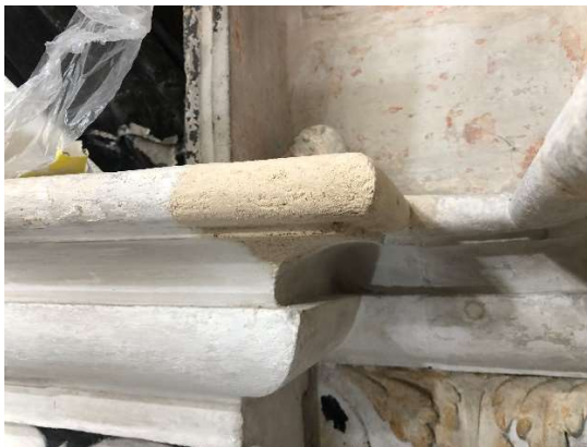
Figure 47 Completed repair to the sinister main mantle
