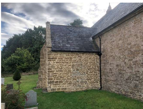
Figure 11 New pointing on the west wall
