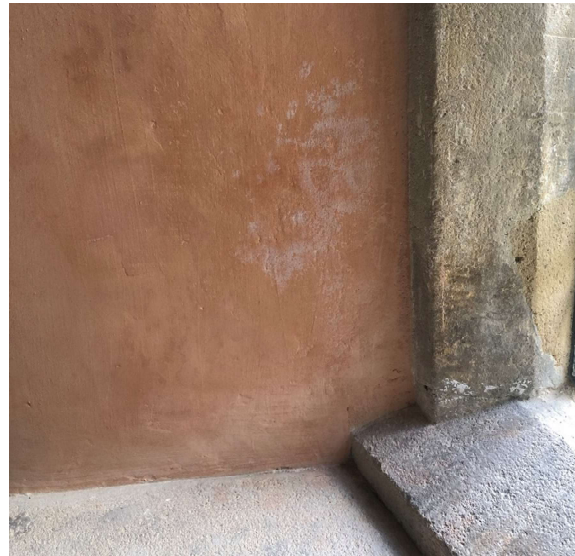
Figure 84 Salt formation on original lime plaster over the new limewash north corner of window; September 2022
