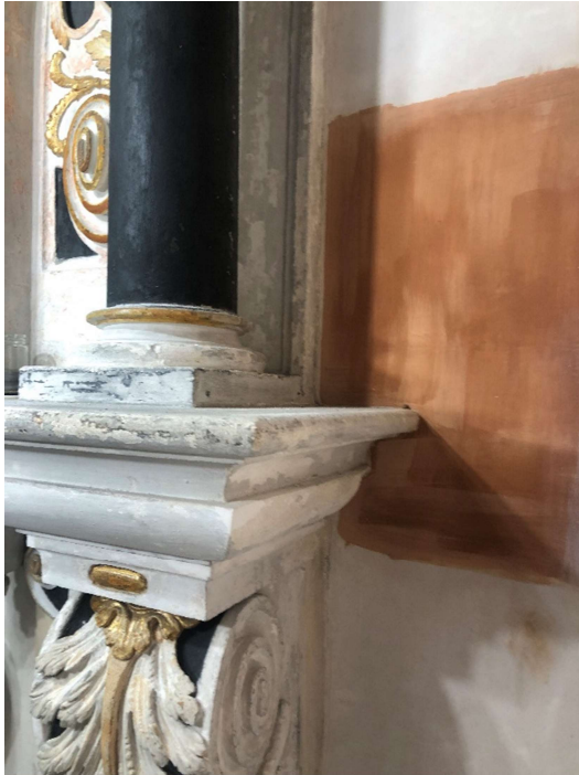
Figure 13 Sample No.1 of the Limewash - Terra Maroc
