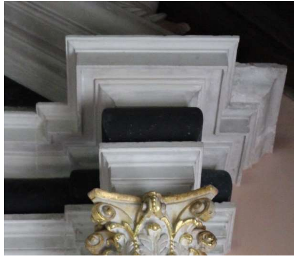
Figure 82 Sinister cornice (after repair)
