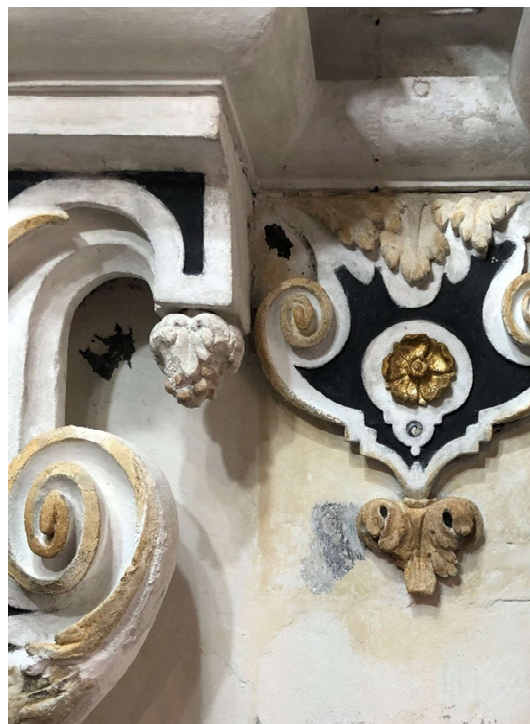
Figure 57 Sinister grape and leaf embellishment fixed in place
