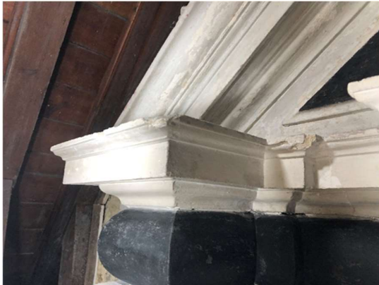
Figure 78 Dexter cornice (before repair)
