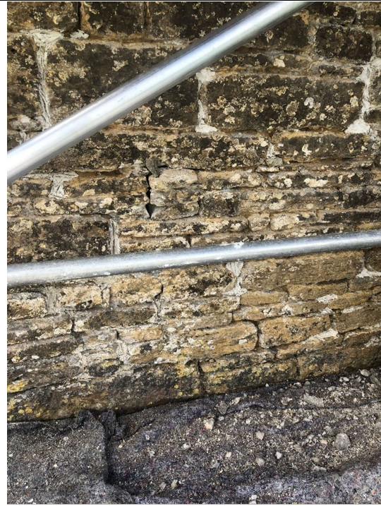
Figure 89 Exterior north-east lower putlog hole
